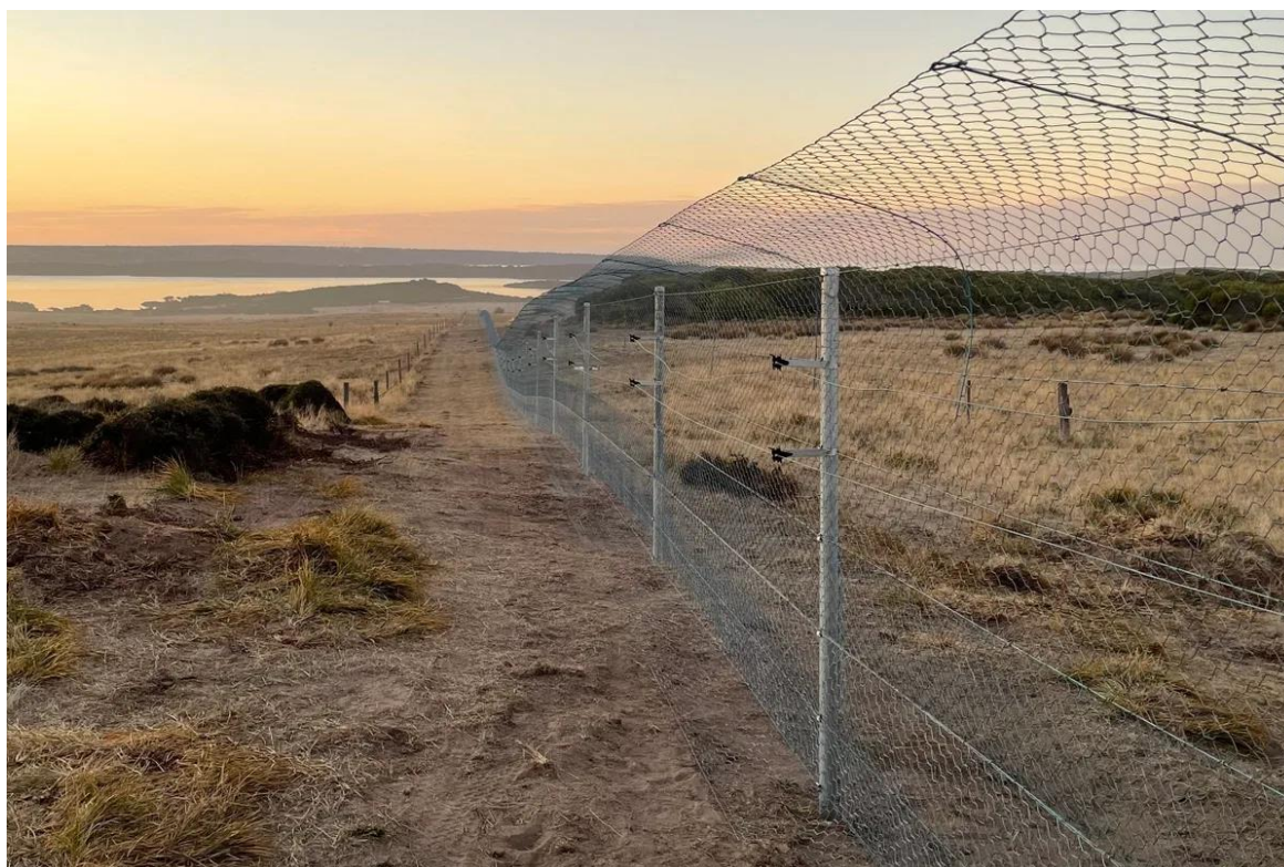
Figure 2-4 Example of a fence designed to exclude feral cats. The photograph shows a 3 km long predator fence across Kangaroo Island, Australia.
