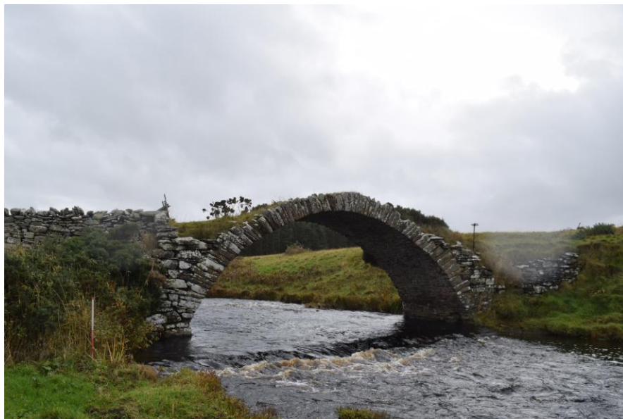
Figure 13-19 Forss Water humpback bridge (ORCA 53)
