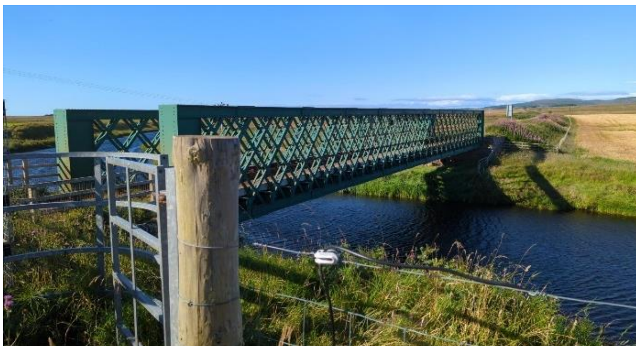
Figure 12-9 Railway bridge over the River Thurso where the Halkirk railside to river link core path ends
