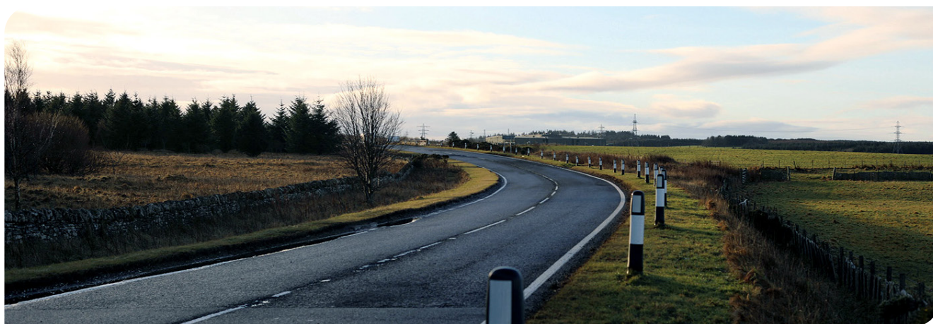
View from Junction of A9, Spittal and to Halkirk © WSP
